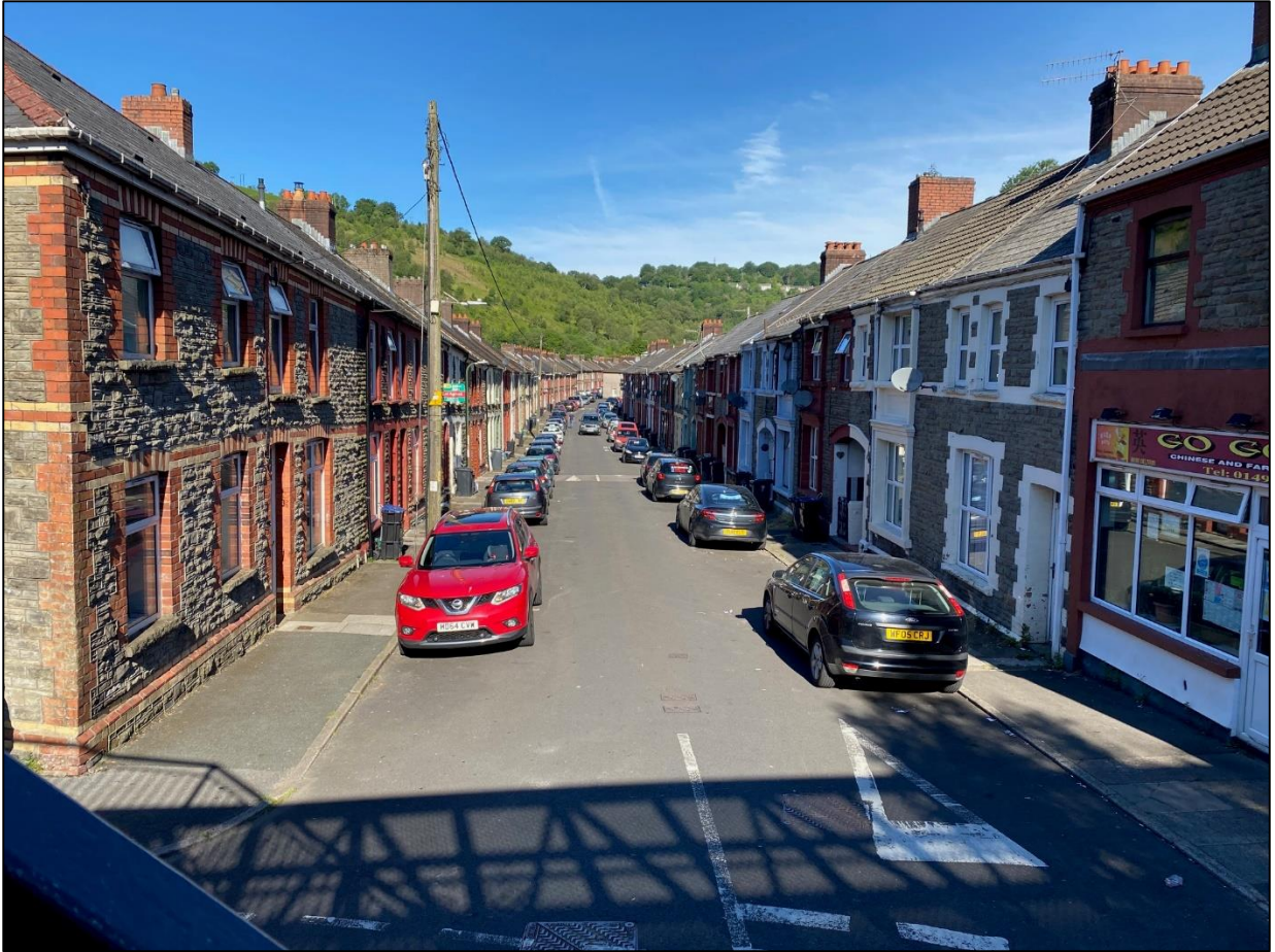
Photograph 6 Photograph Railway Street view West.
