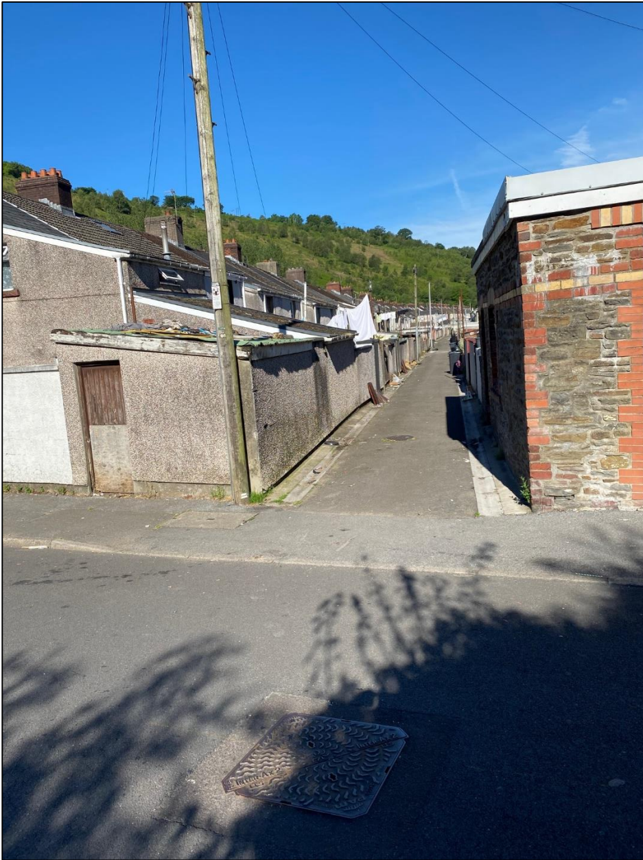
Photograph 5 Rear Lane between Meadow Street and Railway Street. Manhole that was blocked by composite board during Storm Dennis at forefront of photograph. View West. (June 2021)
